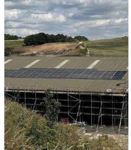
The solar panels being installed at Curzon Lodge Transport Depot
